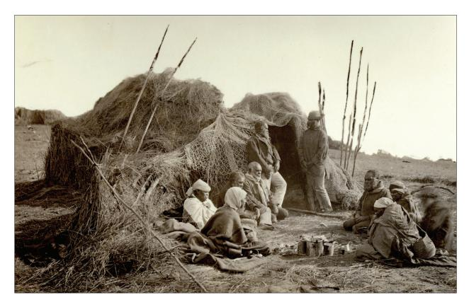
**Figure 1.1.13** A large Ngarrindjeri *ngowanthi* (hut) on the hill overlooking Raukkan (Point McLeay Mission) on the shores of Lake Alexandrina in about 1880. The hut is a solid construction, with a timber frame and a windbreak extension. Fishing nets and spears can be seen. (Photographer S. Sweet, courtesy of South Australian Museum)
